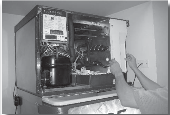
4. Remove evaporator cover.
