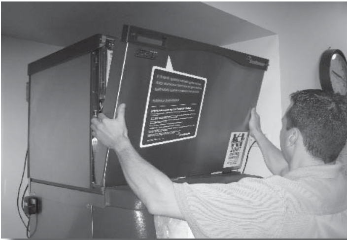
1. Remove front panel
