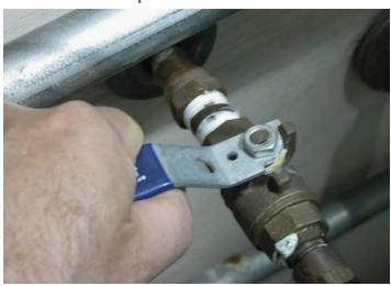
14. Open water valve and remove funnel.
